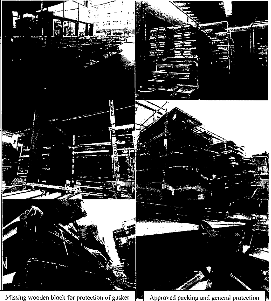
Missing wooden block for protection of gasket
