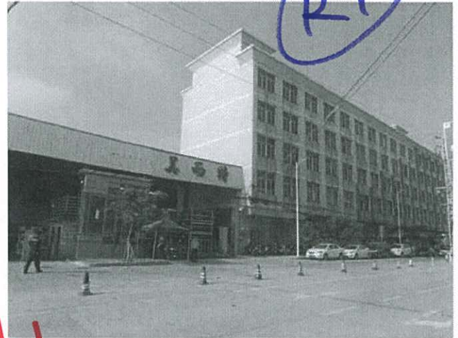
2. General view of Midi Factory
