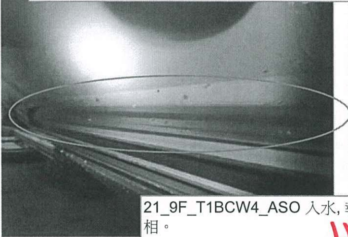
19_Water leakage was found inside spandrel backpan
