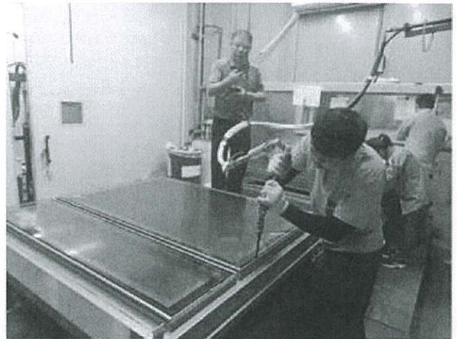
20_Application of Structural sealant
