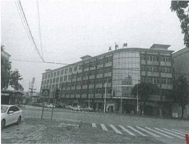
1. General view of Midi Factory
