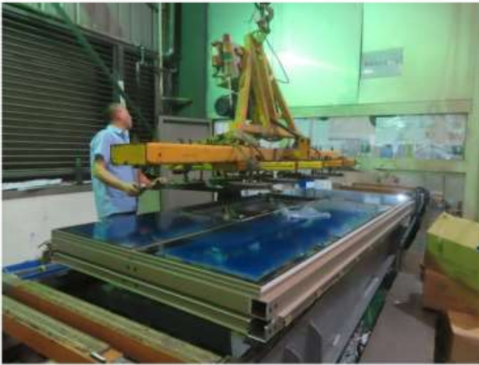
19_Fixing of Glazing
