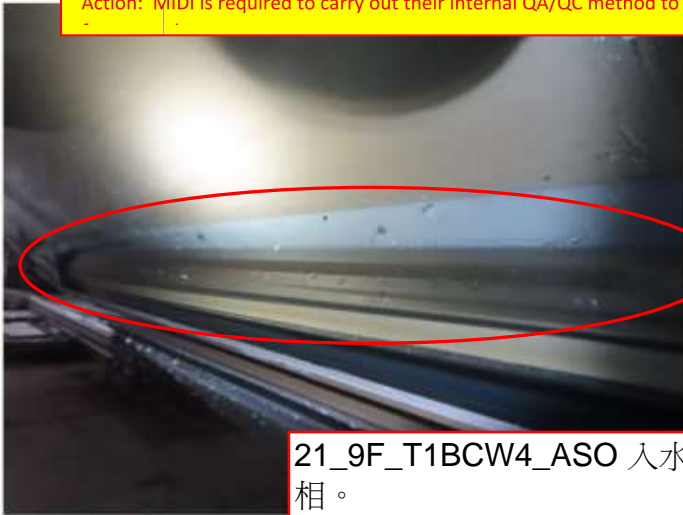
19_Water leakage was found inside spandrel backpan
