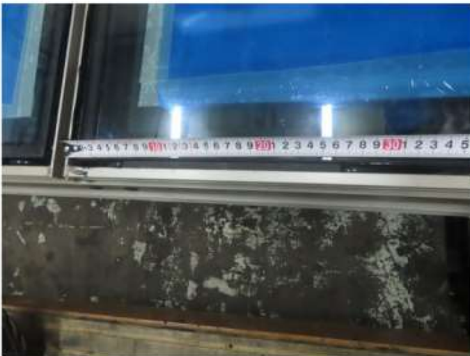
21_Check length and position of setting block
