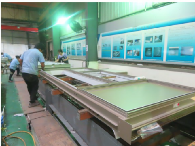
9_Flame cleaning prior fixing of glazing
