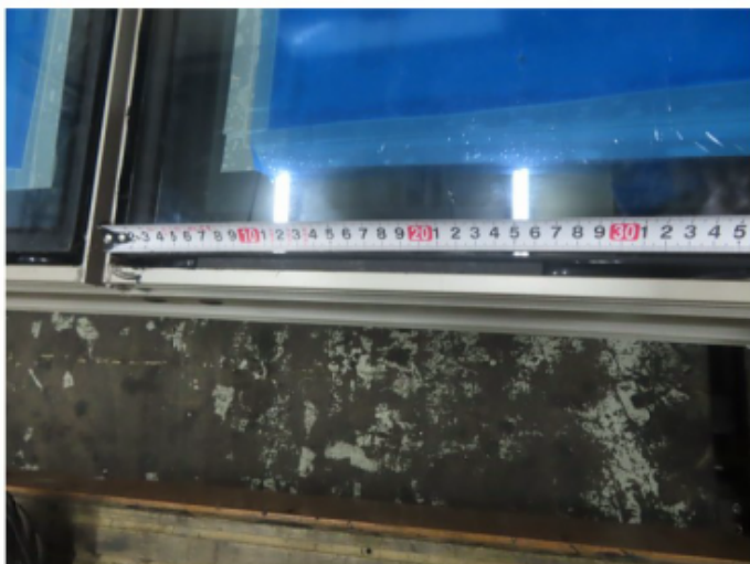
21_Check length and position of setting block
