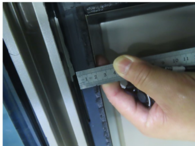
30_ Repair the defect of on spandrel sealant and back pan
