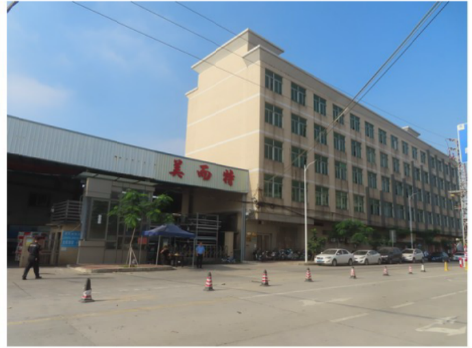
2. General view of Midi Factory
