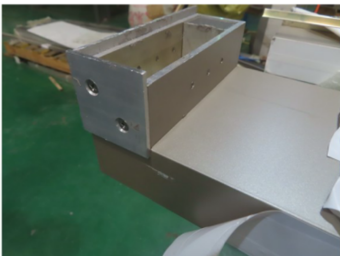
5_Trial assembly of mullion and transom for sliding door
