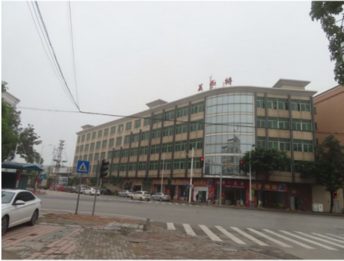
1. General view of Midi Factory
