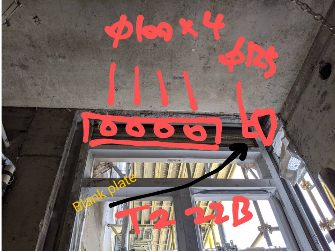
Proposed modification of plenum box
